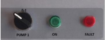
If the fault lamp is energized, the thermal magnetic switch has opened the circuit. If the thermal magnetic switch is constantly opening the circuit, the pump is consuming too much current, or the current setting is wrong. In this case, the situation should be reported to the authorized service.
